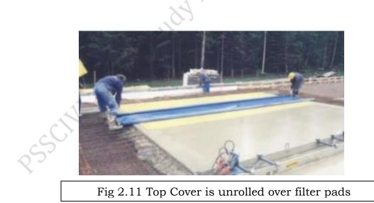
After compaction by surface vibrator, filter pad is placed leaving all sides. The top cover is then placed on the filter pods and rolled out till it covers the strips of exposed concrete on all sides.
