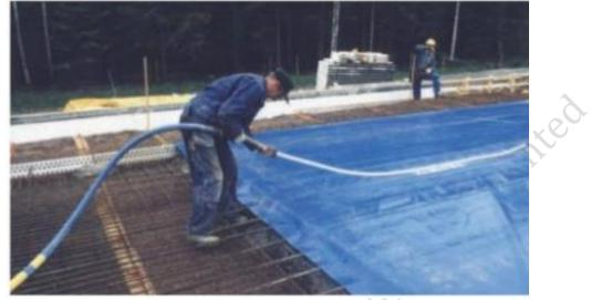
Fig 2.12 Top cover is connected to the suction of the vacuum pump. It is important to check that top cover seals against the fresh concrete outside the filter pads
