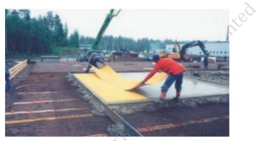
Fig 2.10Filter pads are placed so that there will be a sealing edge around the entire filter pad surface
