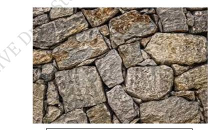
Fig 1.1 Rubble Masonry
