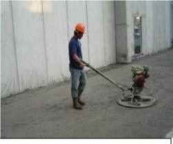
Fig 2.6 Using Floater Machine
