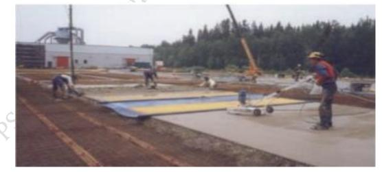
Fig 2.13 While vacuum is on, surface that has already been vacuum dewatered is floated with a power trowel fitted with a disc.
