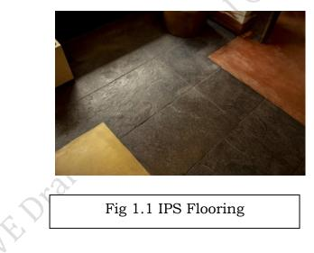
Thickness of the IPS flooring can be decide the as per the requirement of work; in residential floor 75 mm floor thickness is sufficient whereas industrial floor thickness should be kept 150 mm.
